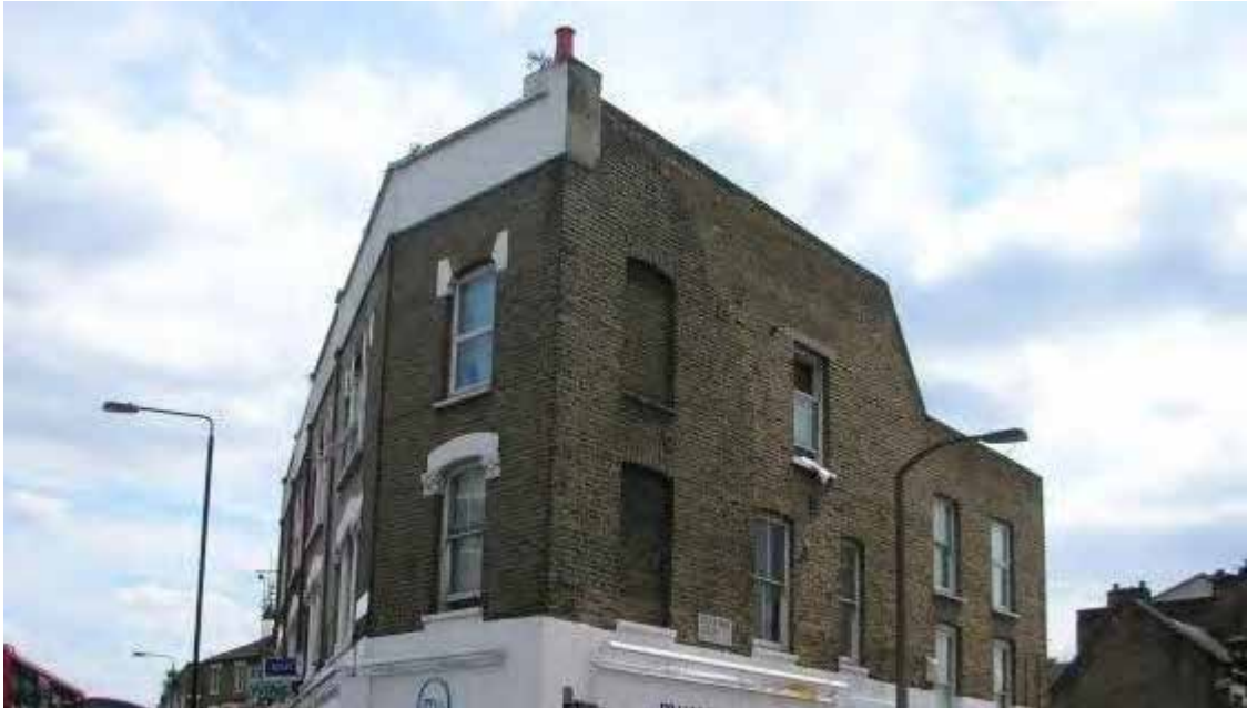
No. 92 Stockwell Road follows an irregular building line.
