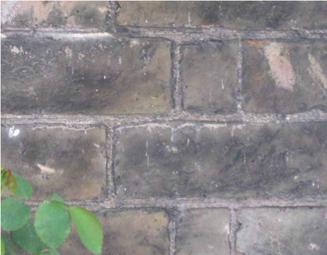
Penny struck pointing is created by scoring the surface with a coin—giving added definition to the brickwork.
