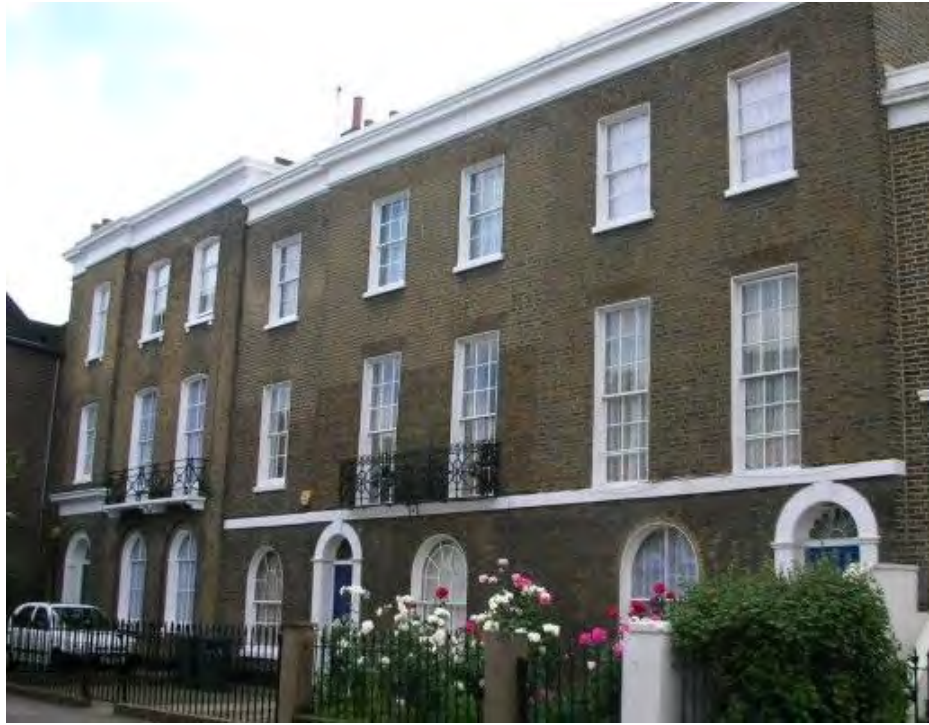
Regency houses on the west side.
