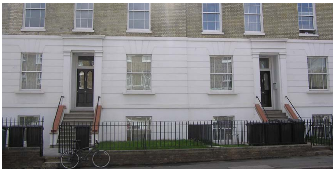
149-155 Coldharbour Lane. An affordable housing scheme by Metropolitan Housing Trust partly funded by S106 commuted payments by developers.
