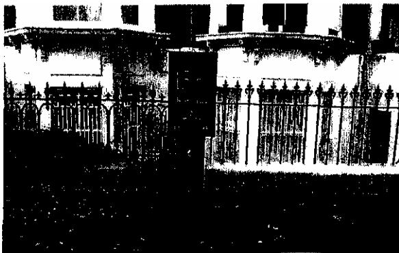
Attractive cast iron railings surround basement areas.
