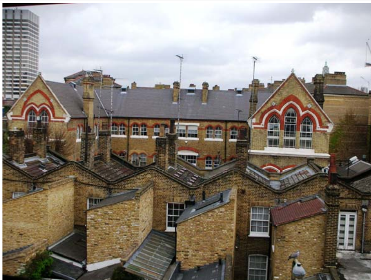
No. 74 Roupell Street (1868) is has yellow stock brick with red brick and stone dressings.
