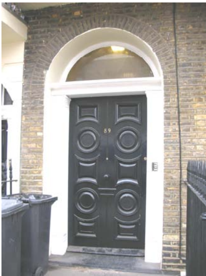
Historic panelled door on Stamford Street
