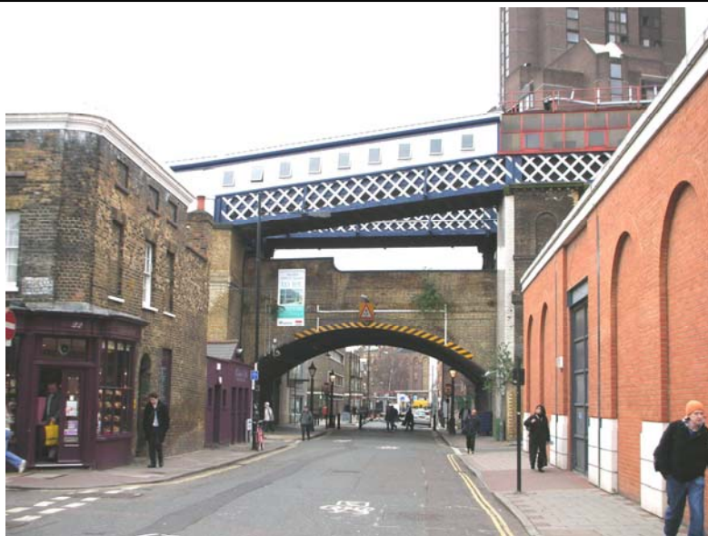
The view South down Cornwall Road is terminated by Waterloo East Station.
