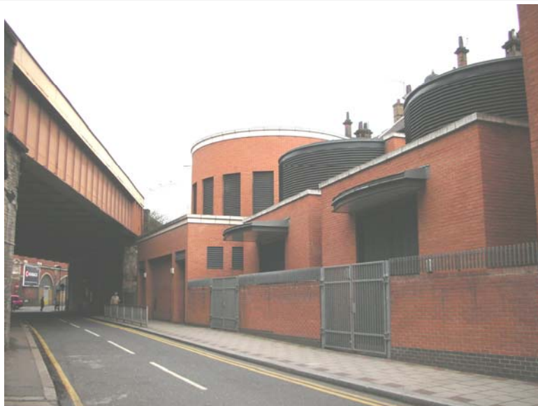
London Underground tube shaft buildings, Alaska Street
