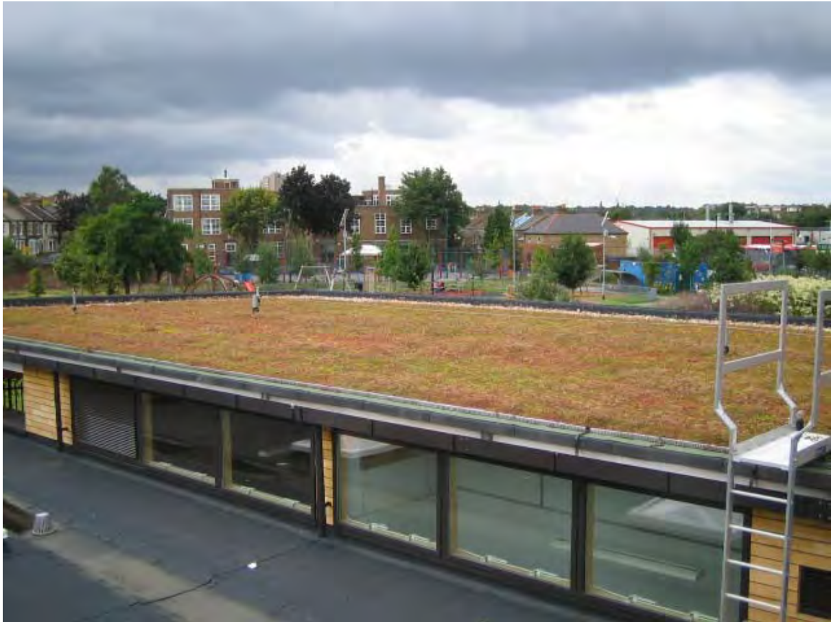
Plate 18. Part of the living roof on the Michael Tippett School, Herne Hill, which is still one of the largest green roofs on any school building in Greater London
